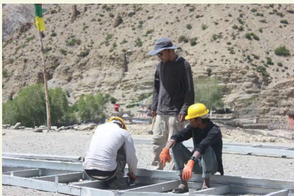
Suman Rai(engineer) and experts working on truss.
