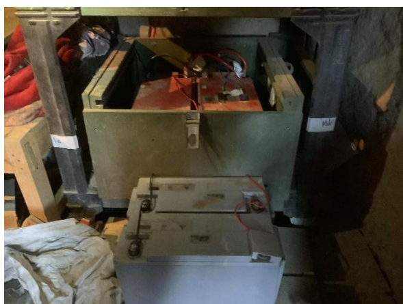
Two 100 AH new battery at power house
